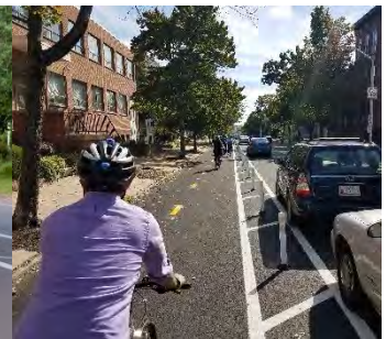
Physically Separated Bike Lane
